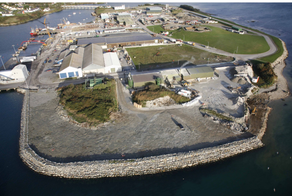
Castletownbere Fishery Harbour, County Cork.
