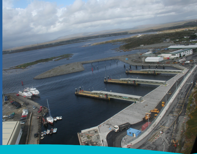
New ferry terminal for Aran Islands, Rossaveel, County Galway.
