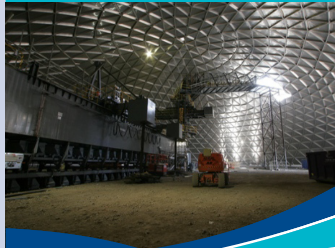
Irish Cement Plant, Platin, County Louth - Limestone storage building.
