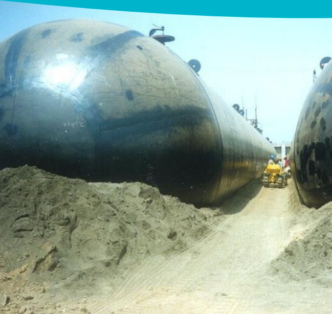
LP Gas storage facility, Usar, India - Mounded storage construction.
