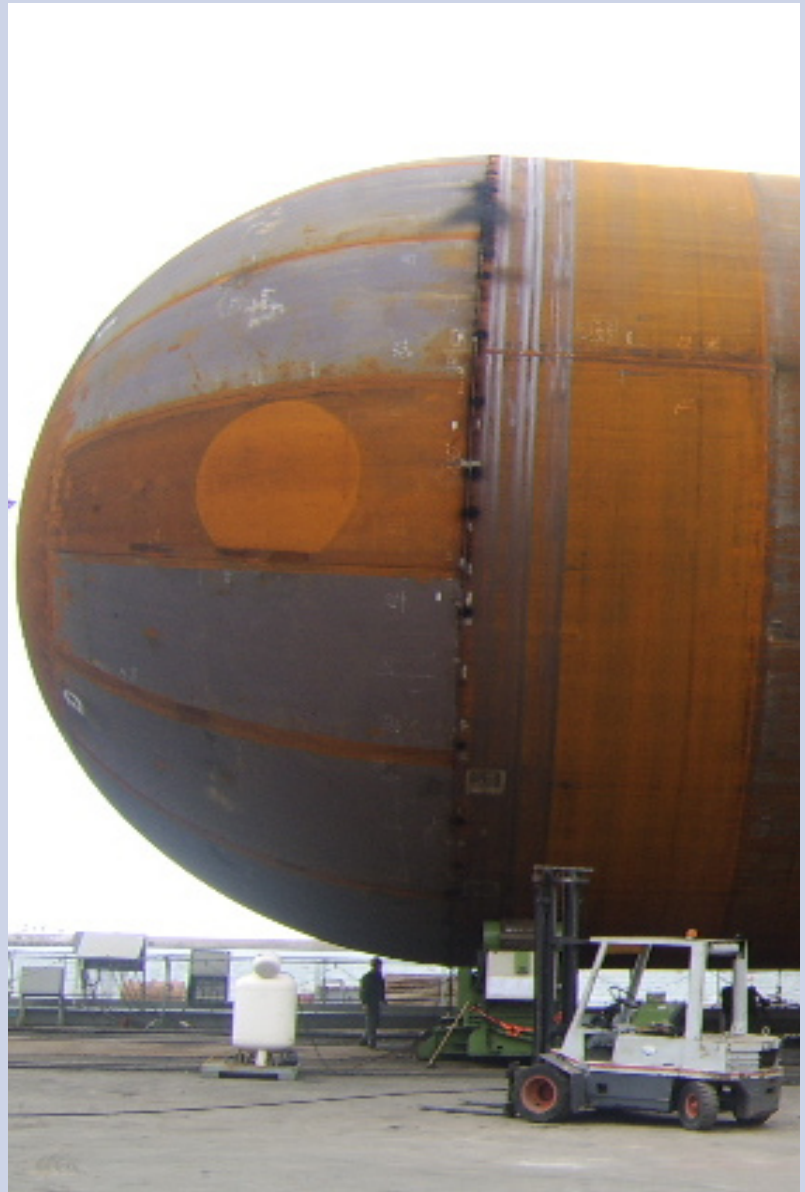
LP Gas terminal, Mauritius - Tanks being fabricated in Italy.
