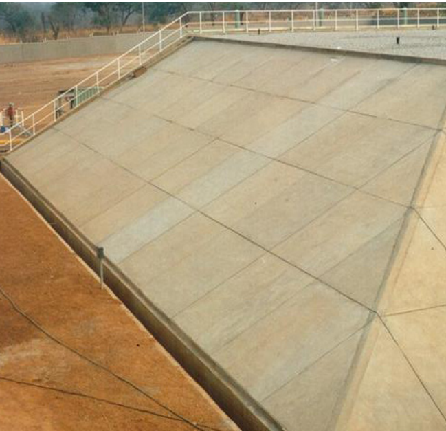
LP Gas facility, Ilorin, Nigeria.
