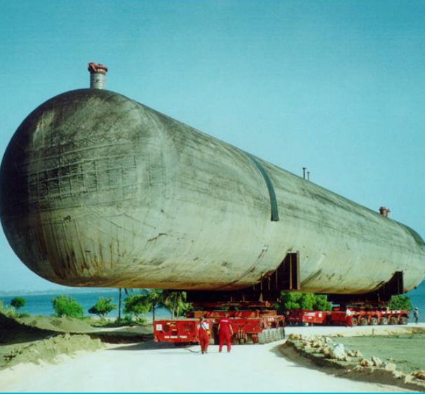
LP Gas import facility, Mombasa, Kenya - tank off-loading.
